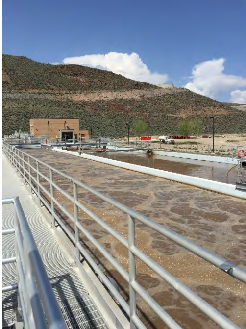
Photo 4.16 - Oxidation Ditches
