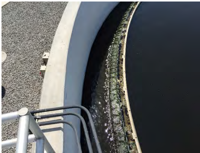
Photo 4.26 - Clarifier No. 2 Launder
