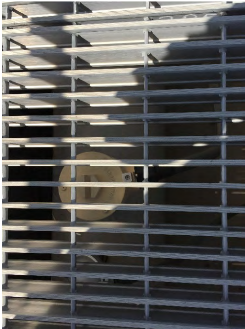
Photo 4.21 - Thermal Mass Air Flow Sensor
