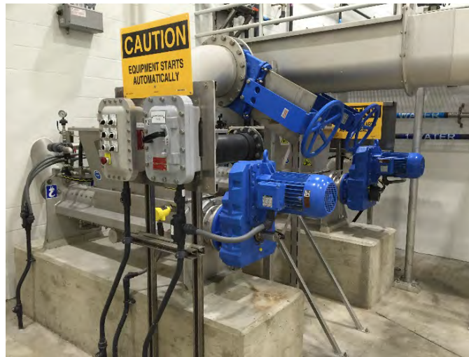
Photo 4.11 - Washer-Compactors
