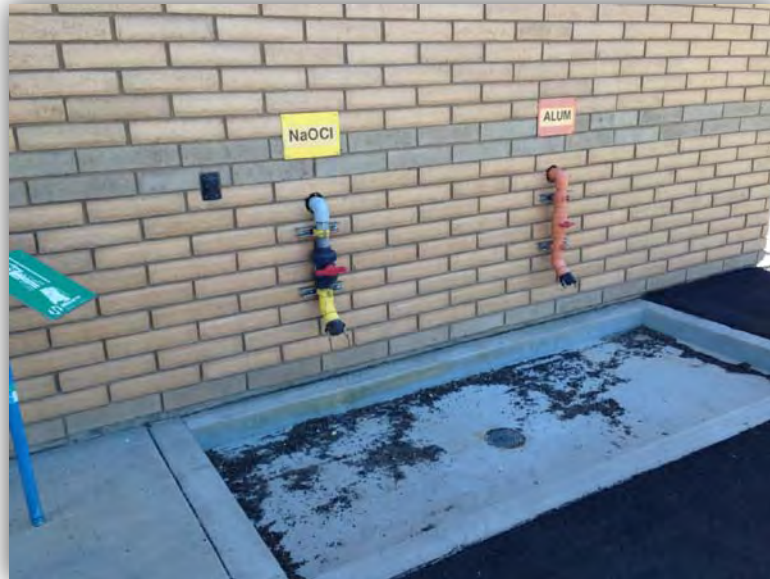
Photo 1 CSB Bulk Delivery Area
