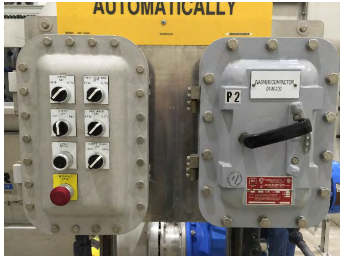
Photo 4.12 - Washer-Compactor LCP
