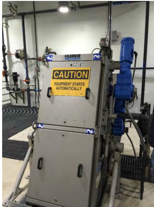
Photo 4.8 - Mechanical Screen
