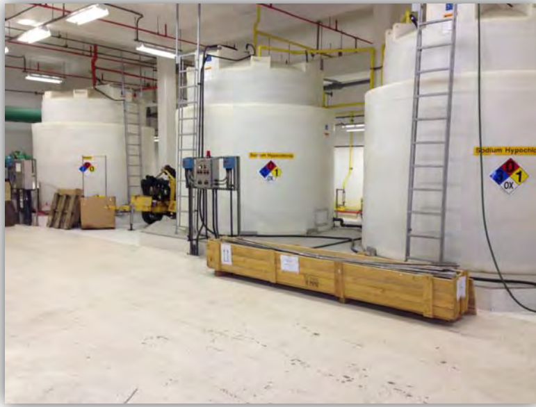
Photo 3 Sodium Hypochlorite and Alum Tanks
