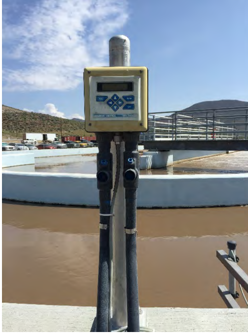
Photo 4.18 - Dissolved Oxygen Probe and Meter
