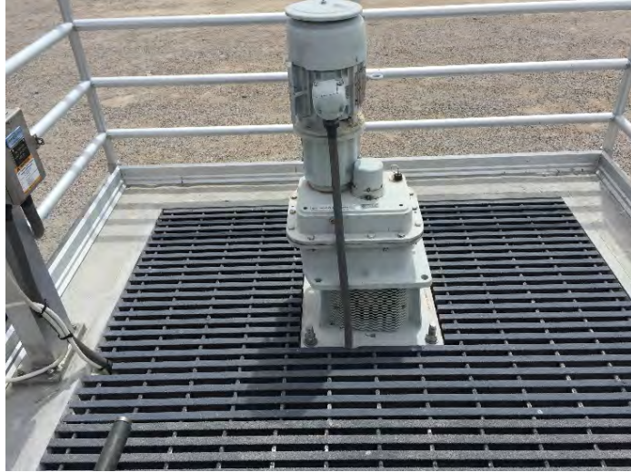
Photo 4.30 - Tertiary Filter Rapid Mixer
