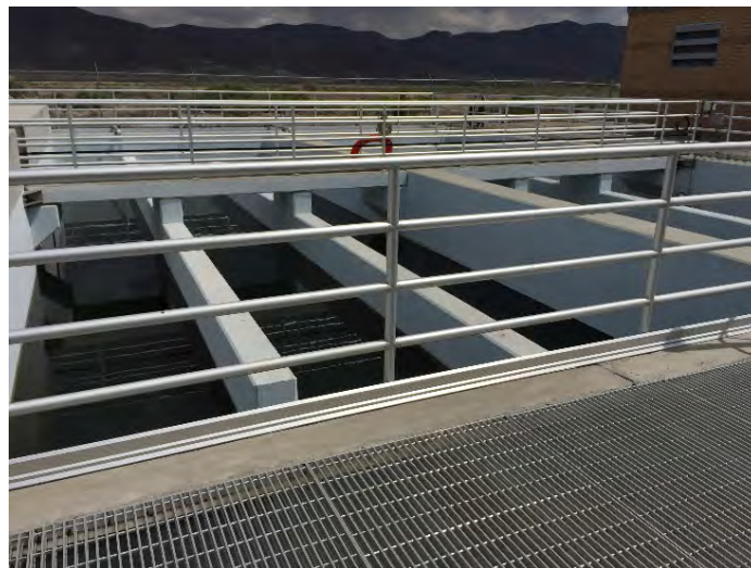
Photo 4.38 - Chlorine Contact Basins
